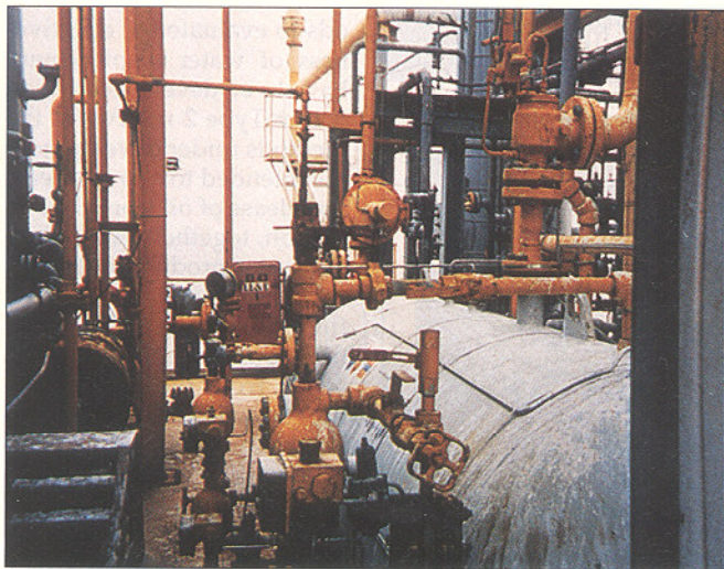
Maintenance costs for cleaning and repainting this production equipment have increased because of paint deterioration from seagull droppings (Fig. 1).
